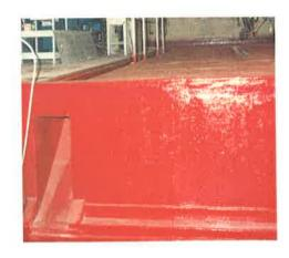
Spillway in an FRP covered floor which directs chemical flow to the run-off trenches. The workmanship required for this detailed work is only achieved with experienced FRP laminators.
