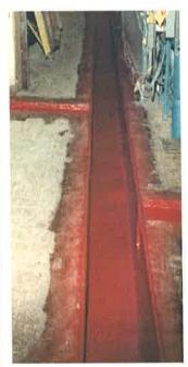
Trench which directed flow in a process chemical run-off was covered with 0.167" tk. FRP. The top recess of the trench was retained so that an FRP Non-Skid Grating can be safely placed over the opening.
