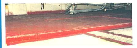
FRP non-skid corrosion resistant covering over an existing concrete floor in a process area. Troughs and walls were covered to make an effective FRP containment area.
